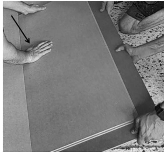
If difficulty to fit panels between each other, check that "fold/down" click system is not damaged or blocked.
