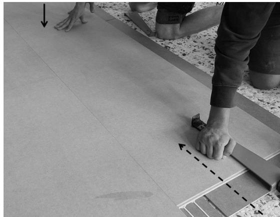
Place the pull bar support against the edge of the lower board so as not to damage the connection system. For a perfect panels fitting, it may be helpful to apply a load located near to the junction of the 2 panels previously installed.
